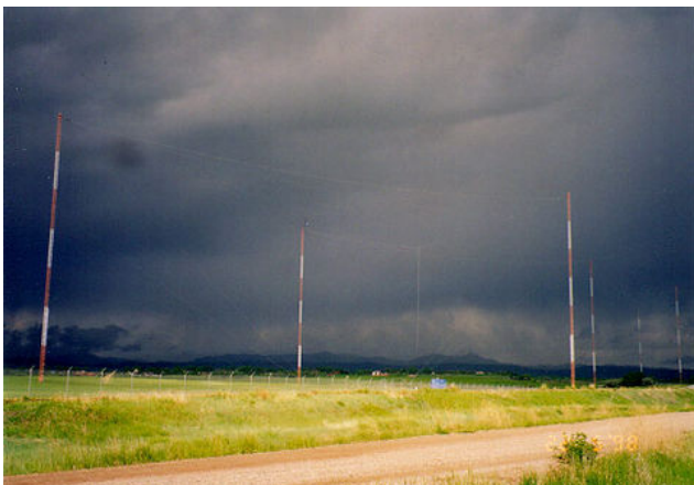
The NIST Radio Station WWVB near Fort Collins, Colorado Photo: NIST
